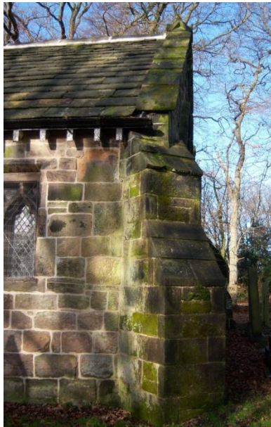
Figure 10 Clasp buttress - south east corner
