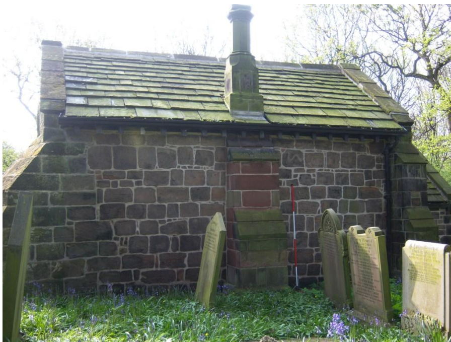
Figure 14 Northern elevation showing chimney, central clamp buttress and lateral buttress at western end
