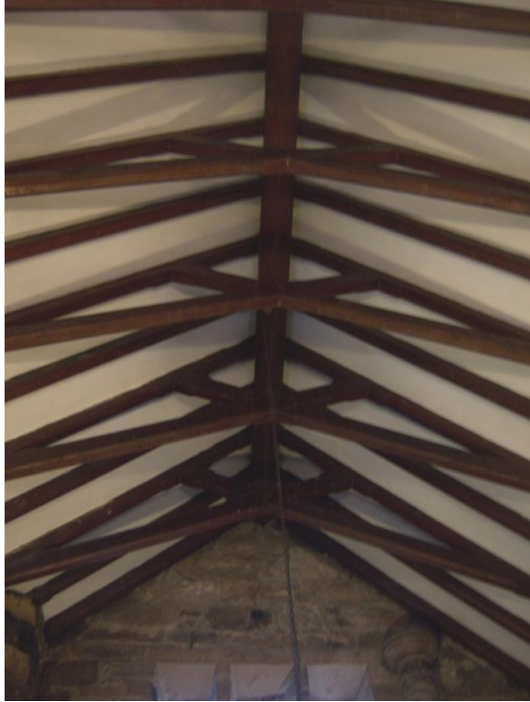
Figure 44 Scissor braced roof of chancel
