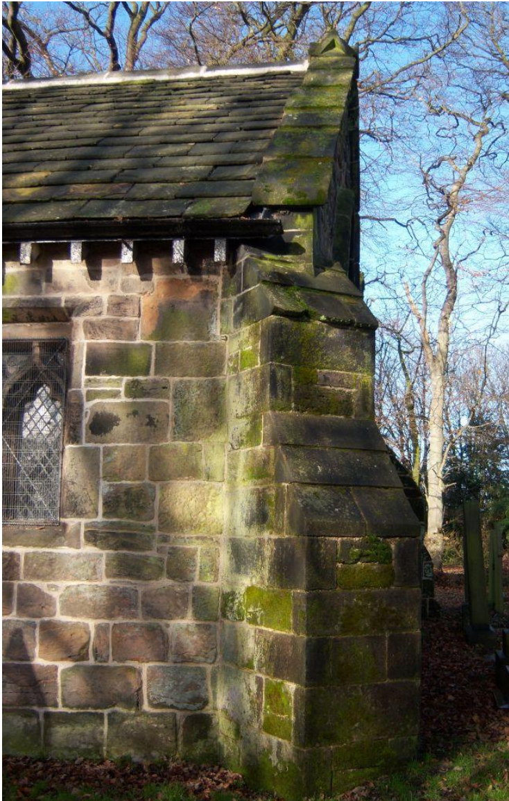
Figure 20 Example of a clasping buttress - south east corner
