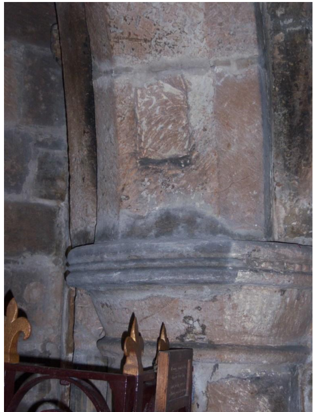
Figure 45 Western respond supporting transitional arcade. Gouge in stone visible above capital - unknown cause
