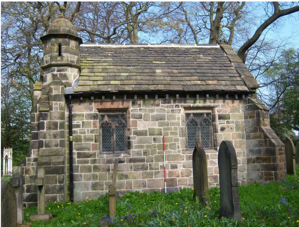
Figure 16 Southern elevation with two windows, each with creped ogee lights. The 19 th century replica can be seen on the left – distinguishable due to a larger lintel
