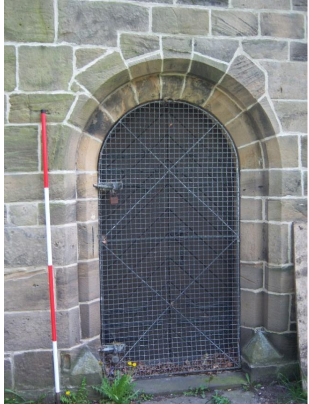
Figure 22 Disused round arched entrance into chancel – western elevation
