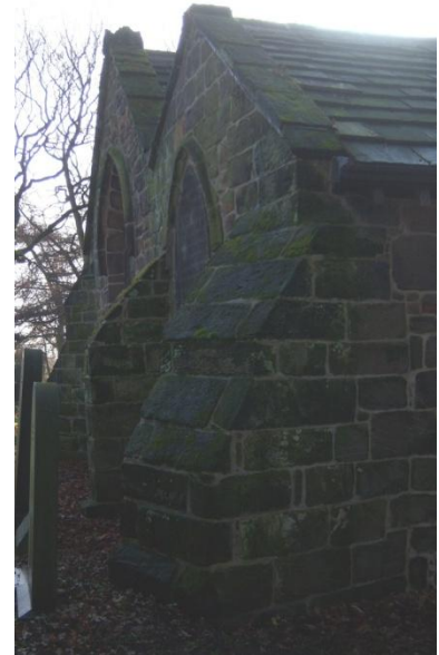
Figure 9 Diagonal buttress - north east corner
