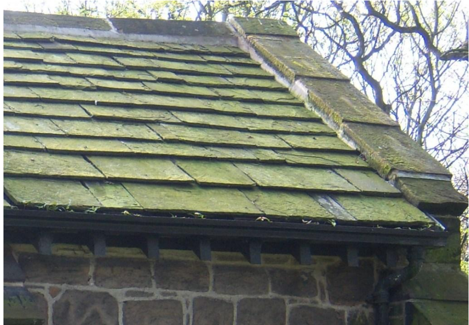
Figure 24 Roof detailing showing stone slating, rafter feet and roof soffit
