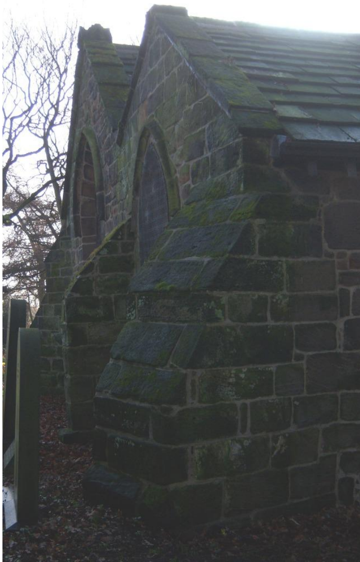
Figure 21 Diagonal buttress - north east corner
