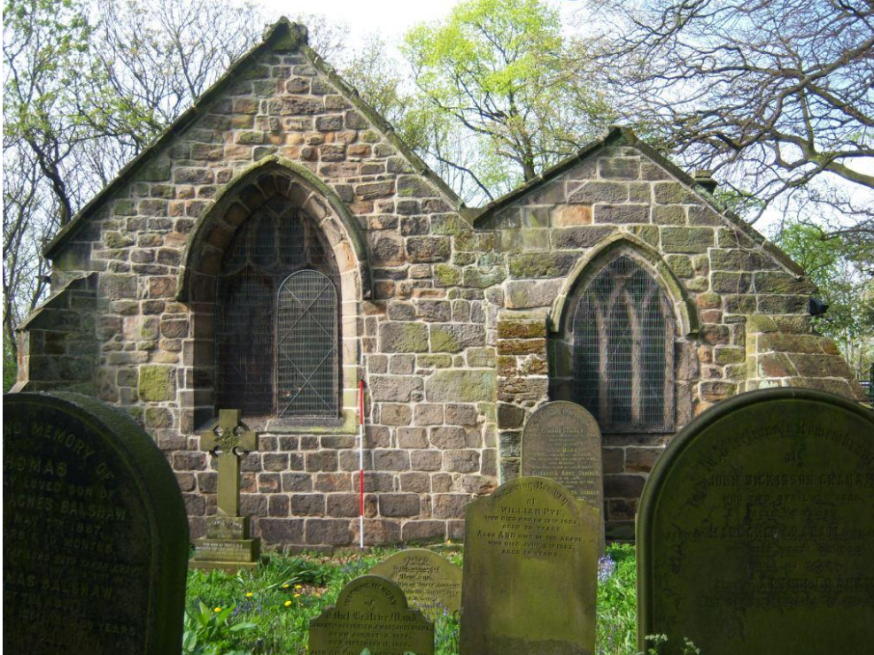
Figure 15 Eastern elevation – also showing the east window of the Unsworth Chapel featuring intersecting tracery
