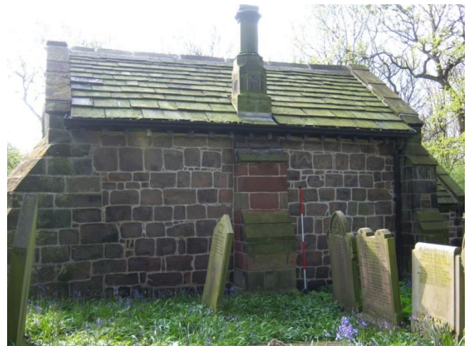
Figure 4 19 th century changes visible in the use of more regular shaped sandstone blocks
